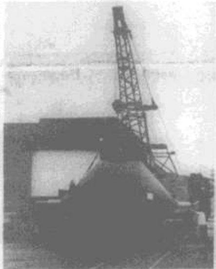
THE 100-TON STEEL UNIT moves slowly along behind the crane as a workman steadies it. The unit was mounted on concrete foundations.
