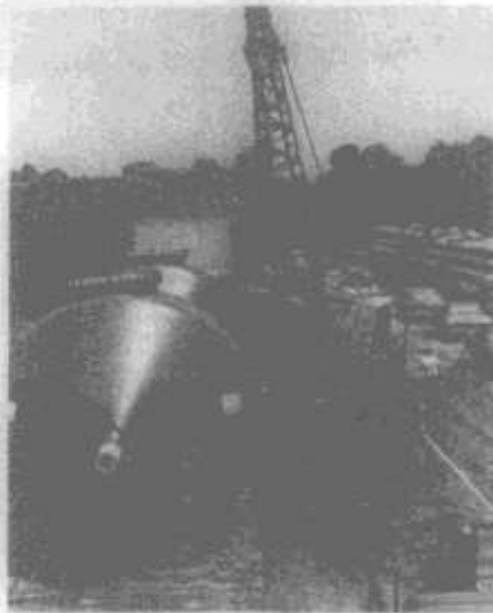
THESE STEEL UNITS, called dischargers, are about 12 feet in diameter, 15 feet long and weigh about 10 tons each. They're in the pulp plant now.
